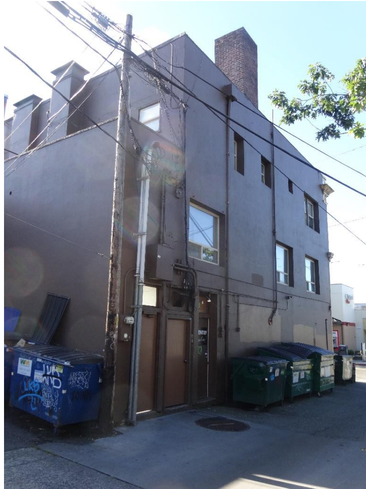
C9: Crescent-Hamm Bldg., northwest corner. Camera facing SE.
