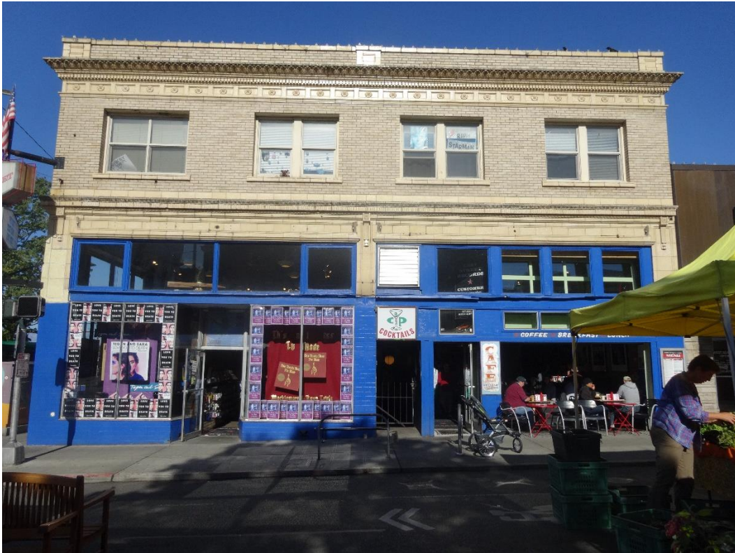
C3: Crescent-Hamm Bldg., east elevation. Camera facing W.
