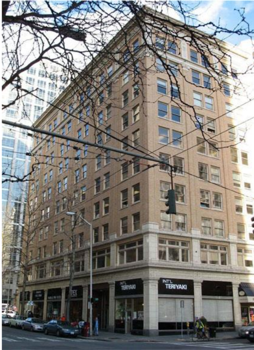
E7: Lloyd Building (1926), 601 Stewart Street. Photo: 2010, Seattle Landmark Nomination.
