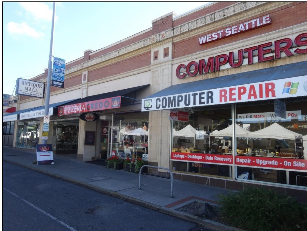
E2: J. C. Penney / Ernst Hardware Building (1926), 4520 California Avenue SW (the Junction).
