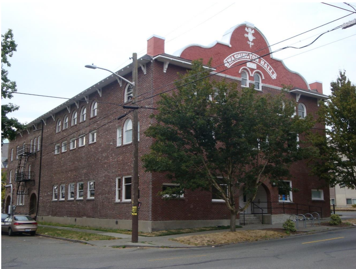
E6: Washington Hall (1908), 153 14 th Avenue. Photographer: Florence Lentz, 30 August 2016.
