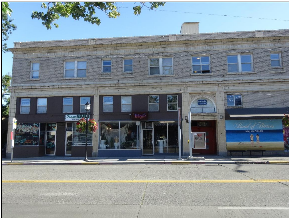
C6: Crescent-Hamm Bldg., south elevation Camera facing N.
