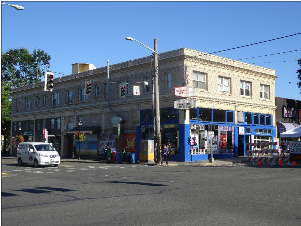
C2: Crescent-Hamm Building. Camera facing NW.
