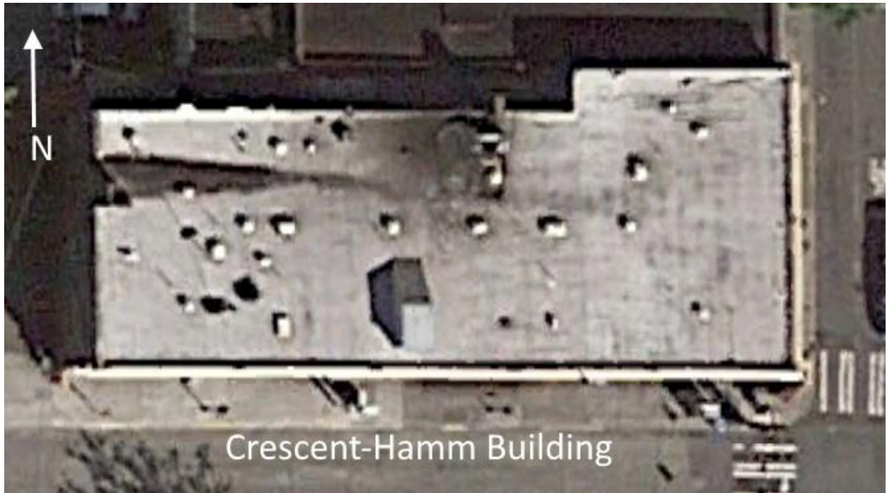
Figure A4: Google Earth Aerial Image, Imagery Date: 4/19/2015 Lat./Long.: 47.561249° / -122.387095°
