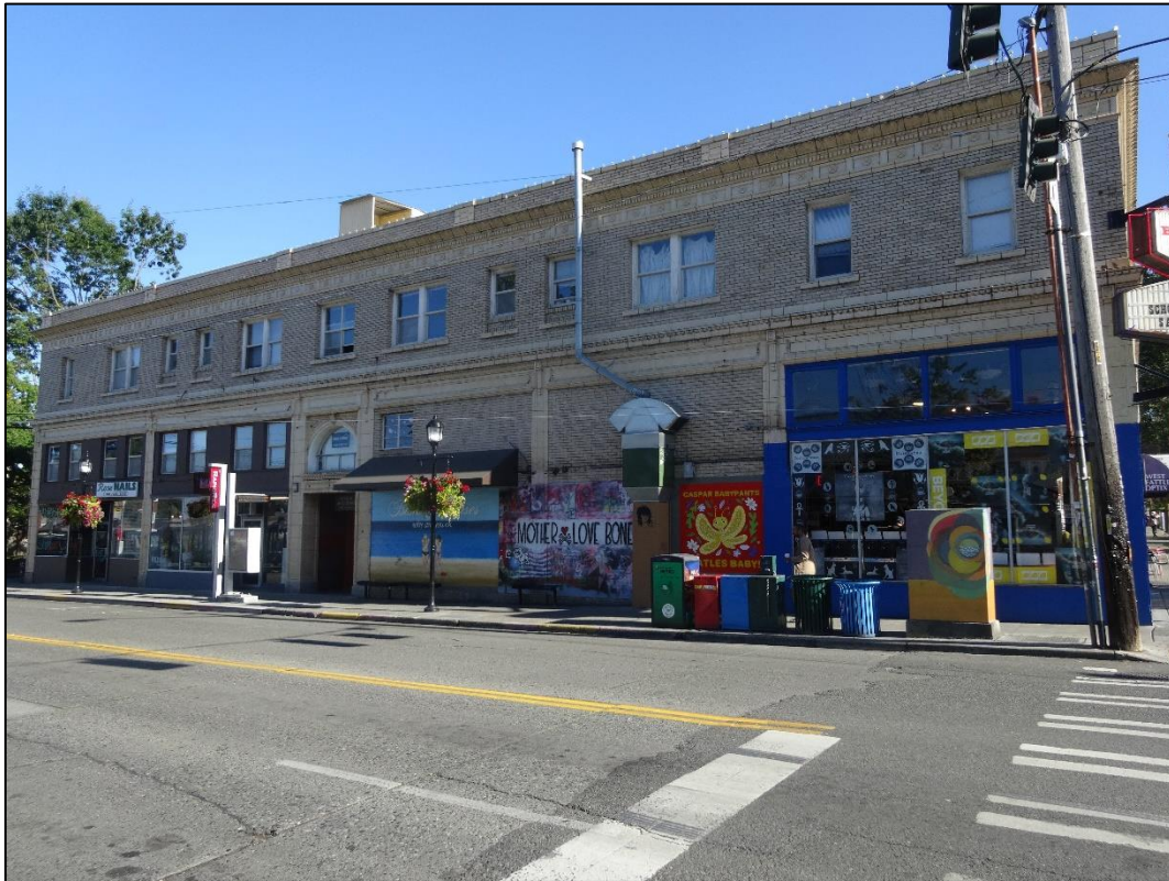
C5: Crescent-Hamm Bldg., south elevation. Camera facing N.
