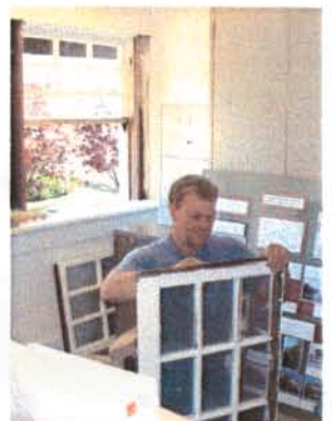
Eric Martin of Johnson Brothers Construction rebuilding upstairs windows.
